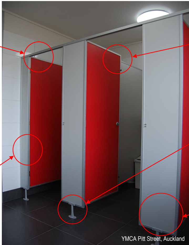
Cast alloy, powder coated pedestal
